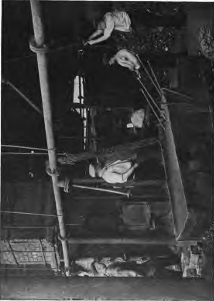
FIG. 15.—Puddling Furnace, Low Moor Ironworks.
